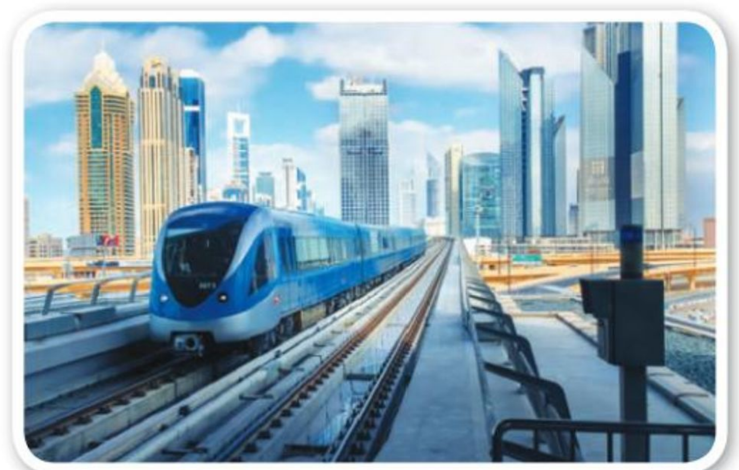
▲ A metro system is unaffected by traffic on the local road network.
